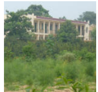
A rural school: overgrown and nearly abandoned.
